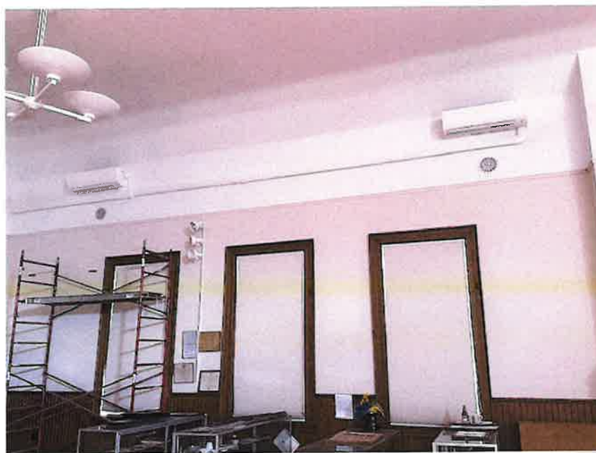
Heat pumps installed on the second floor of Town Hall.
