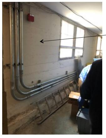
Install 3 inches of closed cell spray foam to the foundation walls full height with a thermal barrier applied to protect.
