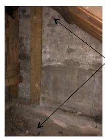
Insulate the foundation walls and install a vapor barrier under the stairs, cut back a section of drywall to access the rim joist.
