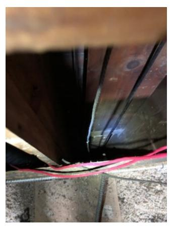
The Attic chase leads to the basement, this chase in the Clock Tower should be sealed using rigid foam and spray applied sealants, no other air sealing should be conducted in the Attic due to presents of Vermiculite berried below the cellulose insulation.
