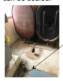
Replace the berried copper line with a coated copper supply line.
