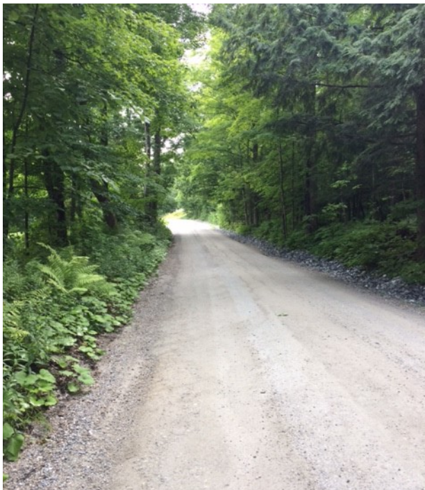
Grader Berm (left) Partially Meets MRGP Standards
