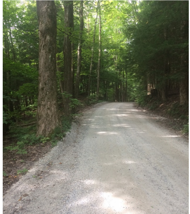
Grader Berm (left) / Eroded Ditch (right) Does Not Meet MRGP Standards
